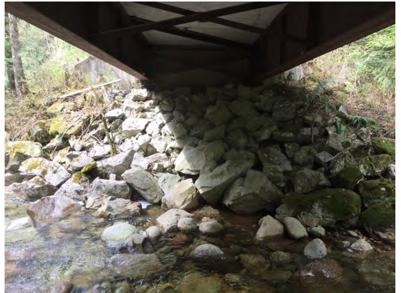
Right Bank Abutment when facing downstream
