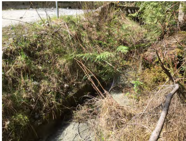
Upstream left bank fill retaining blocks
