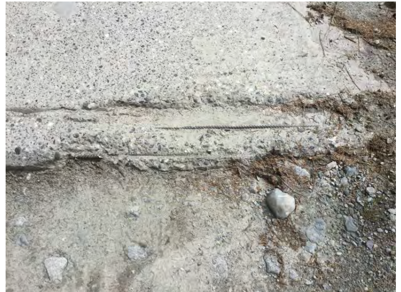
Right abutment top ballast wall condition
