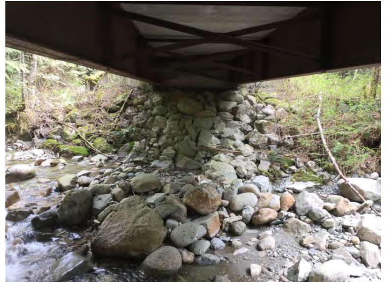
Left Bank Abutment when facing downstream
