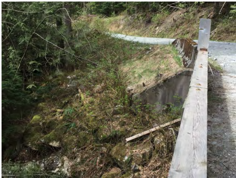
Downstream right bank fill retaining blocks
